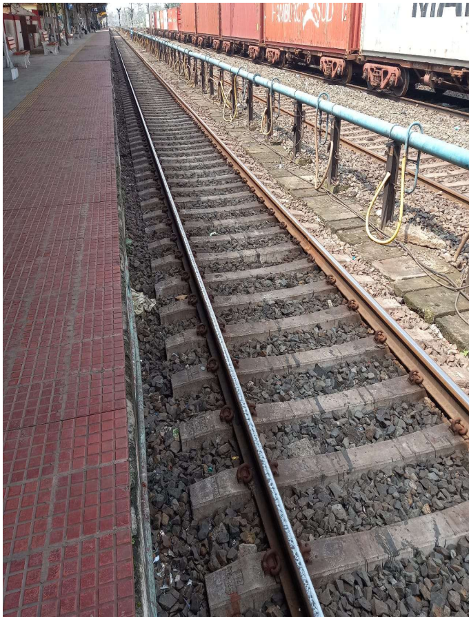
Securing of hydrant pipe at KHARAGPUR Station
