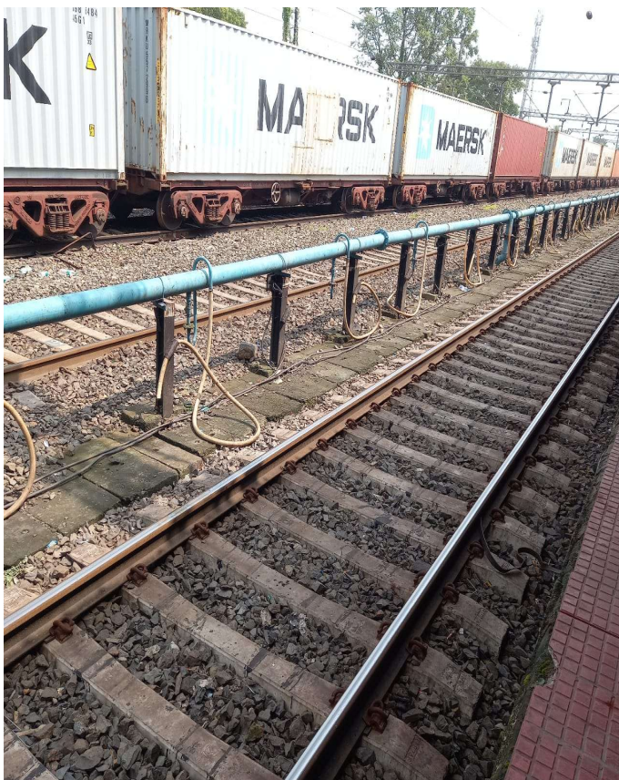
Securing of hydrant pipe at KHARAGPUR Station
