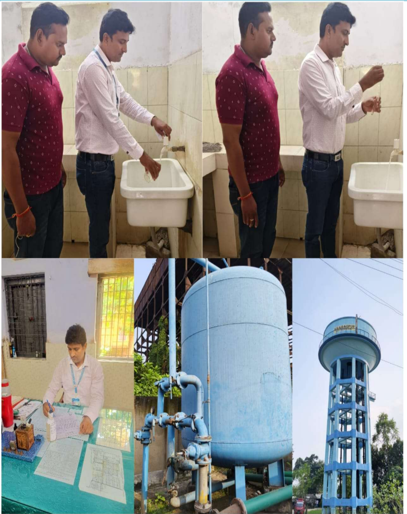
Inspection of water storage tank and filtration plant at Settlement area KGP.
