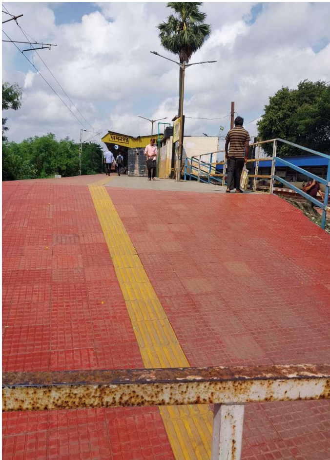
Intensive cleaning of DSNR station
