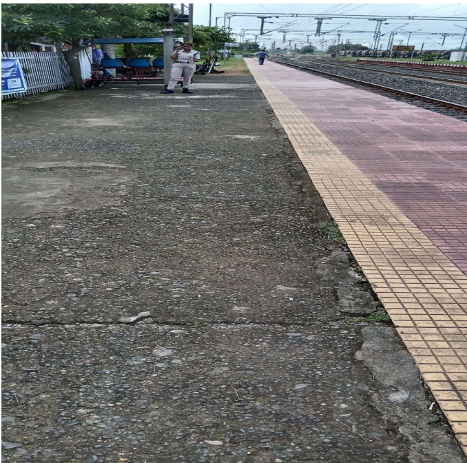
Intensive cleaning of DZK station
