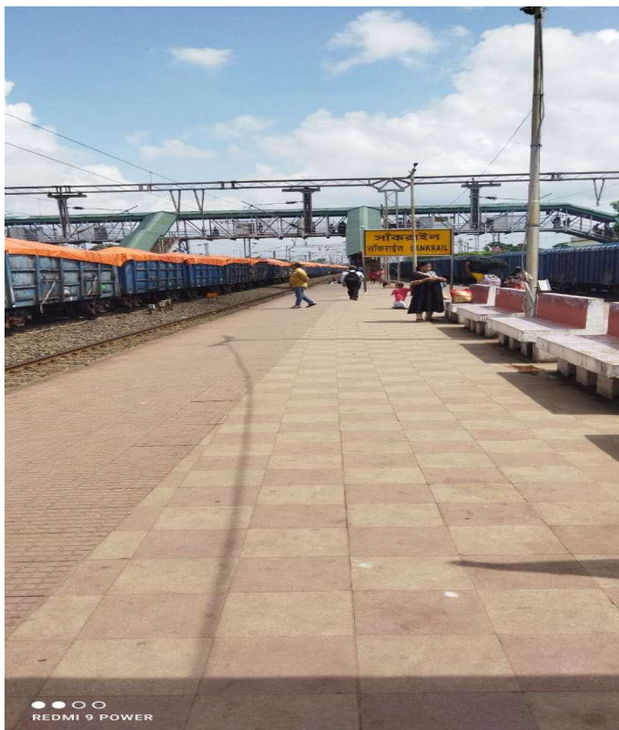
Intensive cleaning of SEL station
