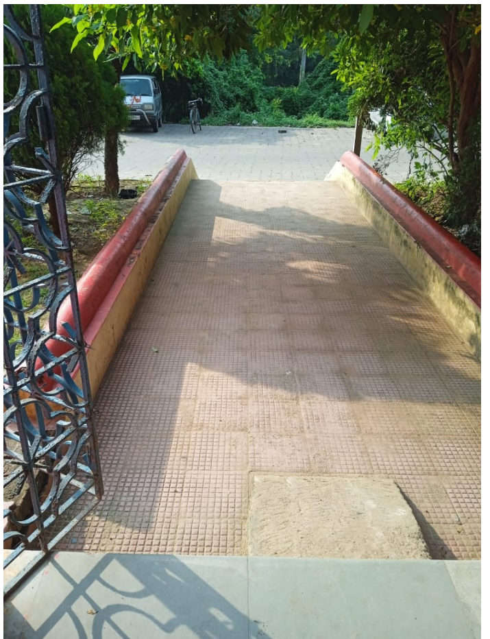
Intensive cleaning at RMRB station
