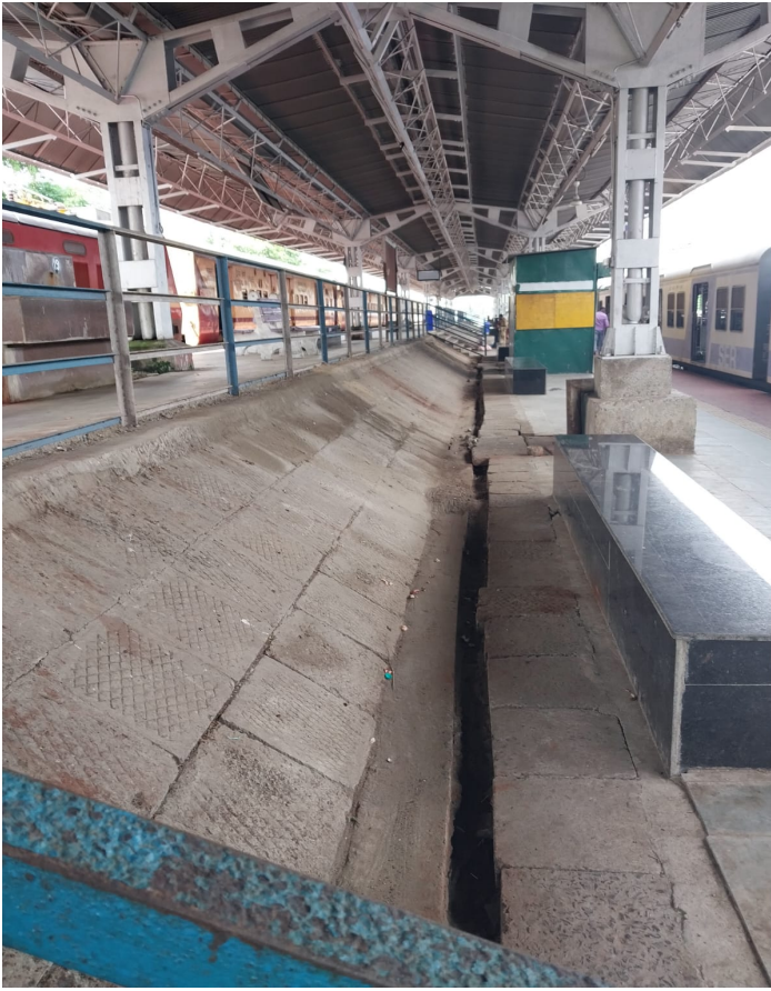
Intensive cleaning at DSNR station
