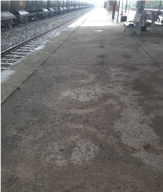
Intensive cleaning of HLZ station
