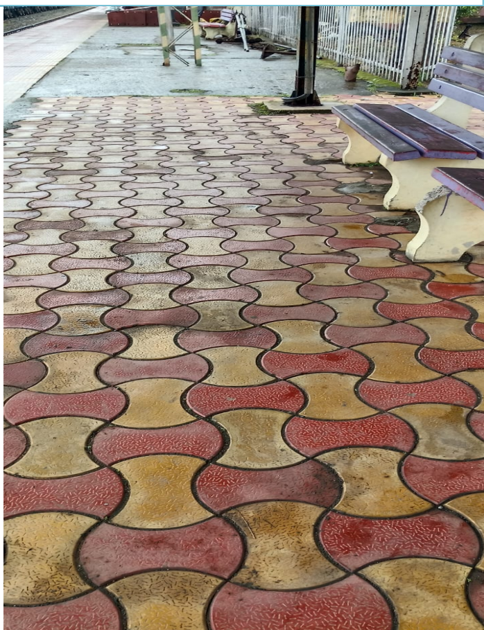
Intensive cleaning of DZK station
