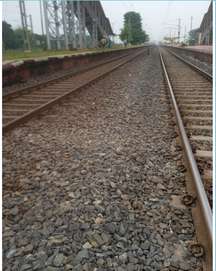
Intensive cleaning at BPE station
