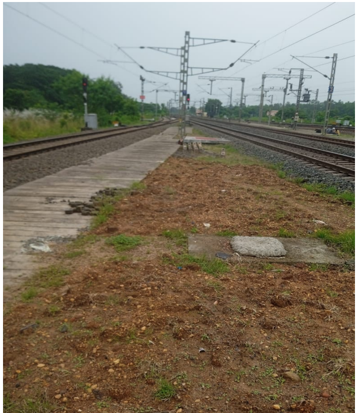
Intensive cleaning of BPE station
