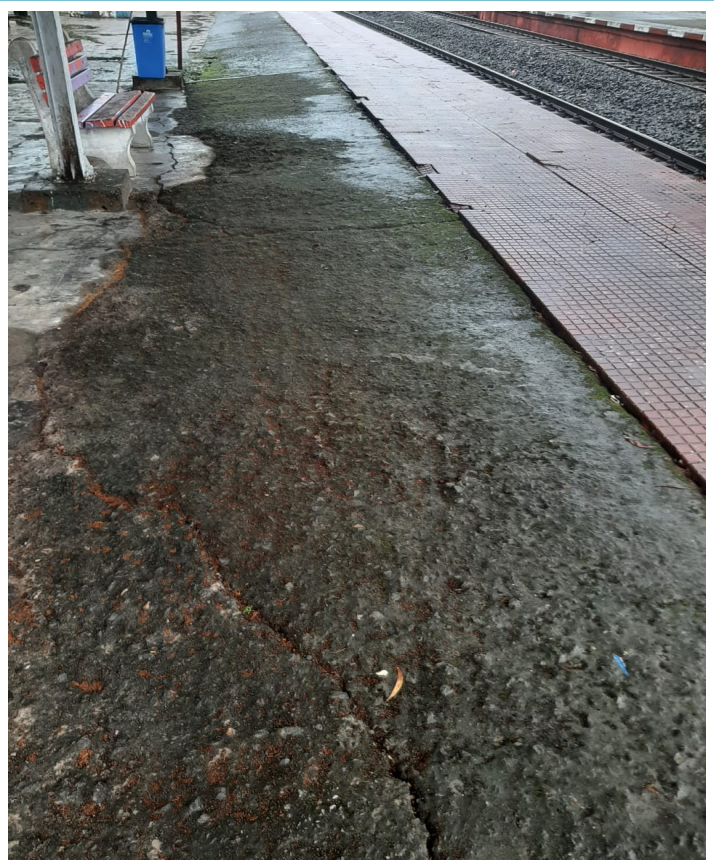
Intensive cleaning of BYSA station
