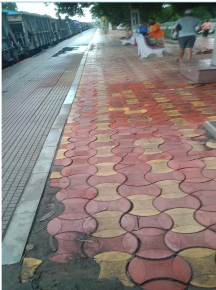
Intensive cleaning of RGA station
