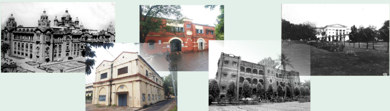
South Eastern Railway Head Quarters (earstwhile BNR) and other heritage buildings in the premises
