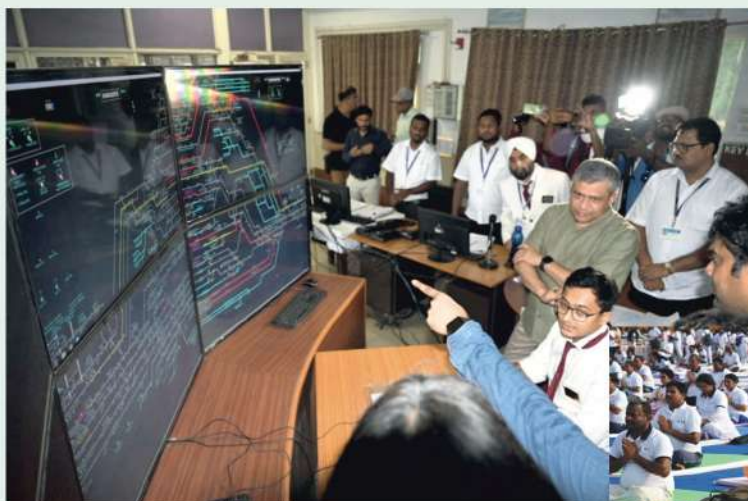
Sri Ashwini Vaishnaw, Minister for Railways inspecting the Route Relay Interlocking (RRI) System at Kharagpur on 21.06.2023.
