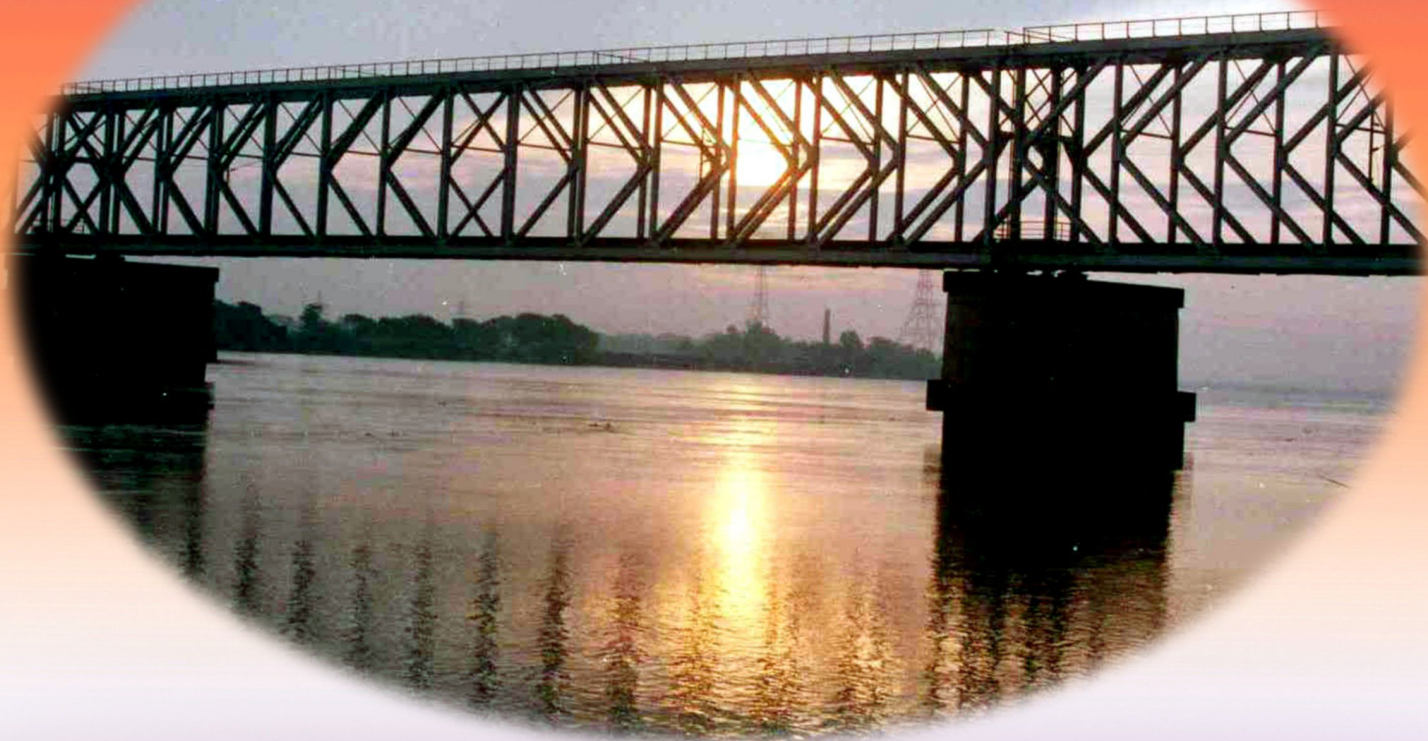
Kolaghat Railway Bridge over Rupnarayan River
