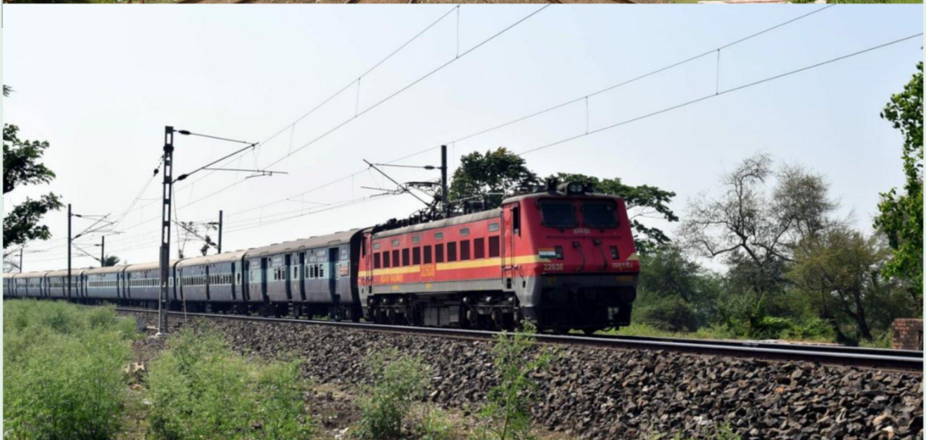
Goods and Passenger Trains are on move in the electrified network of South Eastern Railway
