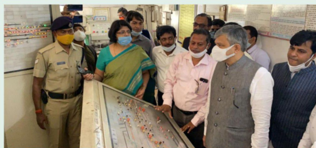
Sri Ashwini Vaishnaw, Hon'ble Minister for Railways, Communications and Electronics & Information Technology inspecting Electronic Interlocking System at Jharsuguda along with Ms. Archana Joshi, General Manager, SER & ECoR on 09-11-2021.
