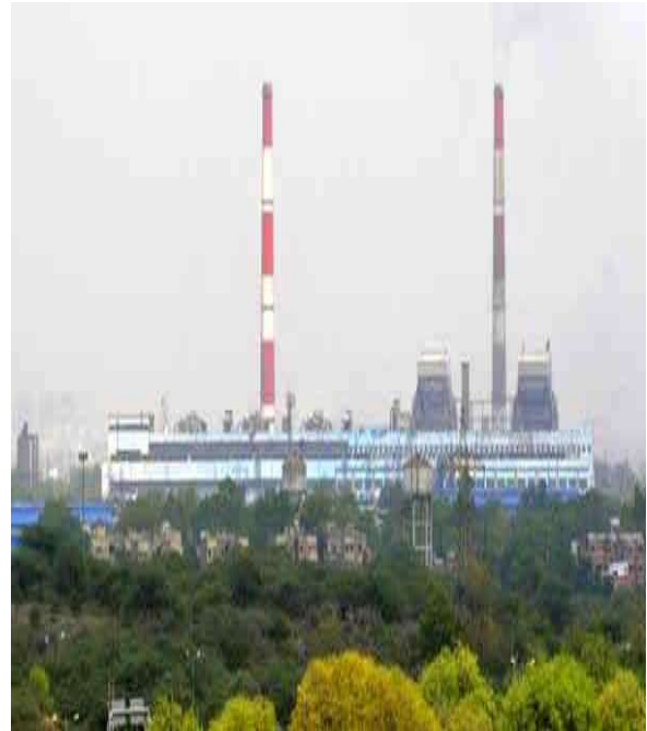
SANTHALDIH THERMAL POWER STATION SANTHALDIH
